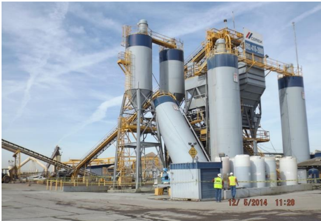
Tower Collapse at 19 th Ave Redi Mix Plant for CEMEX. This occurred while a truck was being loaded
