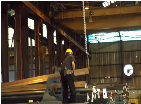
Moving steel beams to be loaded
