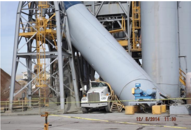
Tower Collapse at 19 th Ave Redi Mix Plant for CEMEX. This occurred while a truck was being loaded
