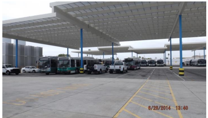
New canopy at the North Yard which was part of the
