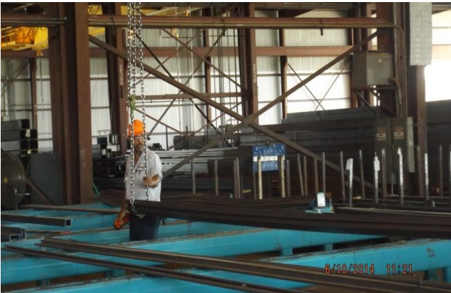
Member moving steel with overhead crane
