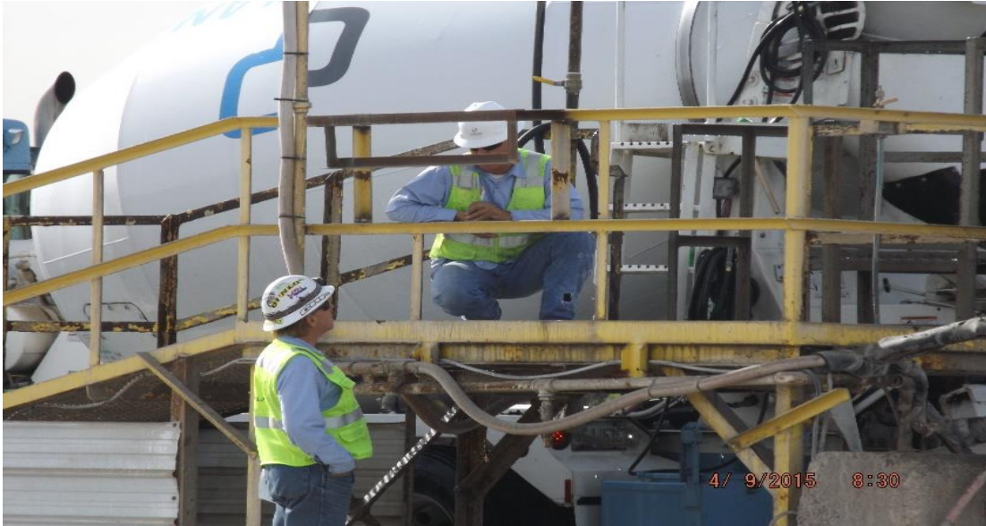
Checking the slump for a load and getting job info.
